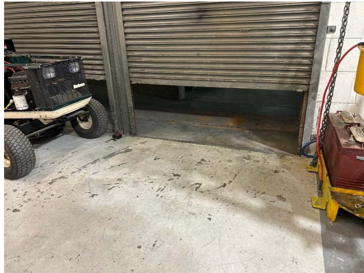
Figure 2 Roller door north wall AG-01 workshop
