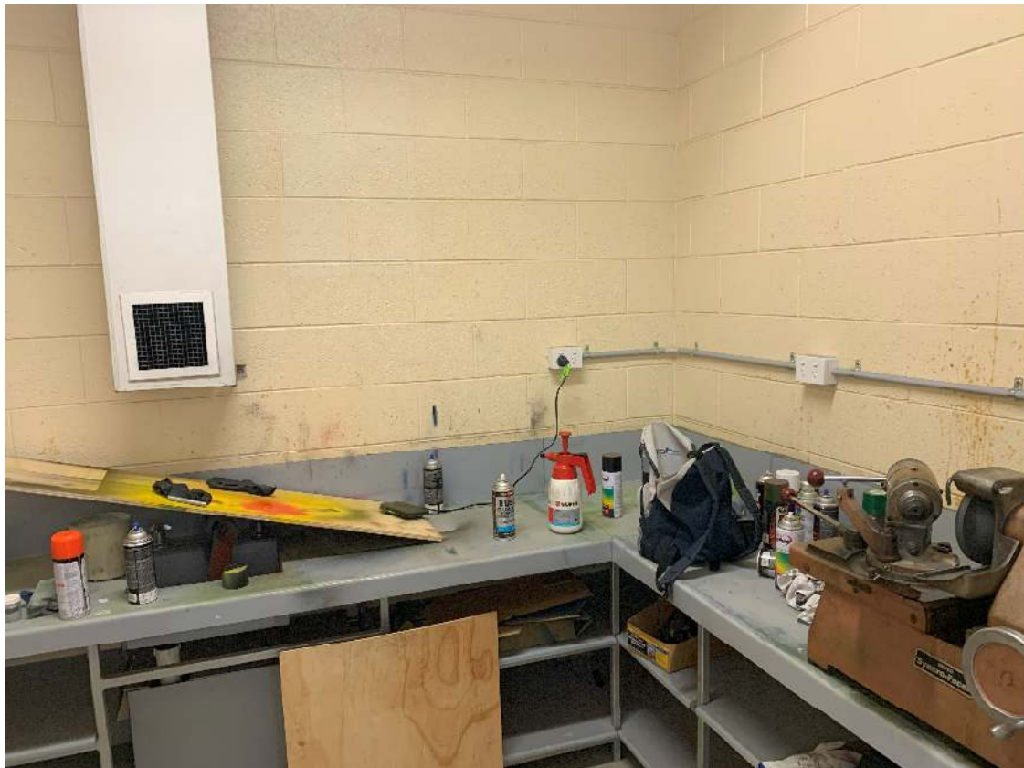
Figure 14 AB-27 Room - Former Battery Storage Area
